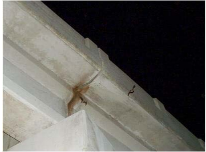
Photo 7: Staining along longitudinal joint. Note guano deposits on the ground. Photo 8: Staining on underside of expansion joint from bat use.
